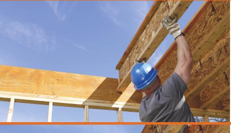
So we engineered our LP SolidStart I-Joists to be 66% wider than your typical lumber joists. That means more stable floors with less bounce and fewer headaches for builders. We're not expecting the Nobel Prize—just strong houses.
